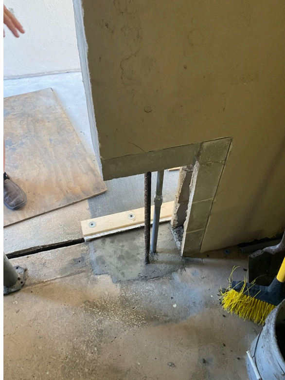
Picture 1: Typical jamb repair
